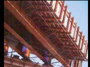
FARRRS bridge beams spanning the East Coast Mainline
